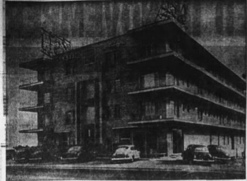
KJLI, GLADWATER.—Radio Station KJLI in Gladewater is owned by the T. W. Lee estate. Its transmitter is in the building at 12 W. Main street and the radio station is on Main street. In addition to the radio station and offices, the building also contains several apartment units.
