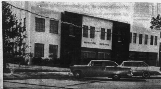
GLADEWATER MUNICIPAL BUILDING
