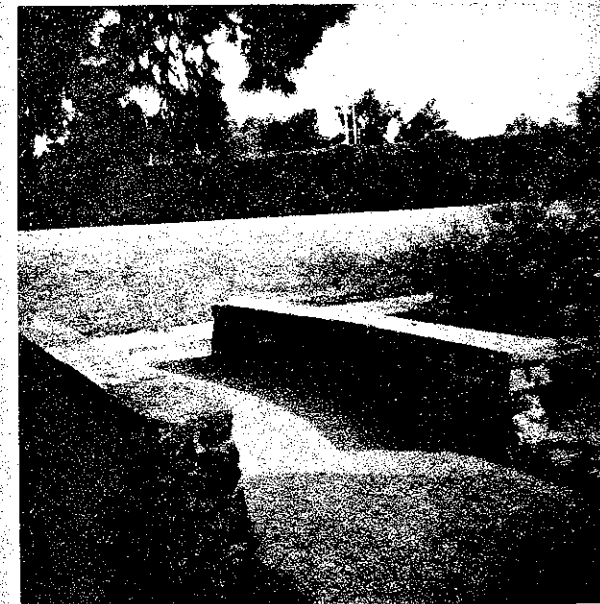
Bridge in City Park 8/11/89
