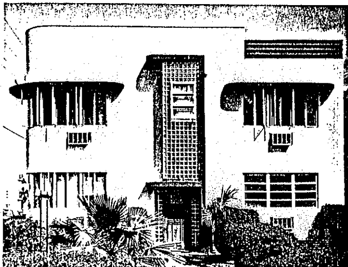
A Michigan Avenue house, Miami Beach, Fla., displays such Art Deco elements as glass brick, horizontal bands of decoration and projecting lintel courses that afforded some respite from the bright Florida sun. (Walter Smalling, Jr.)
