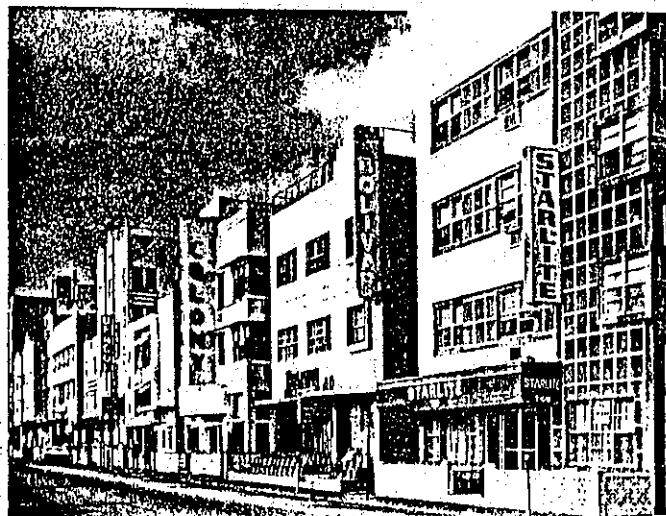
Miami Beach is a treasure trove of Art Deco design. These early 20th-century hotels in the 700 block of Ocean Drive all display various aspects of the style, especially the contrast of smooth-faced walls with details of metal, terra cotta and colored concrete. (Walter Smalling, Jr.)
