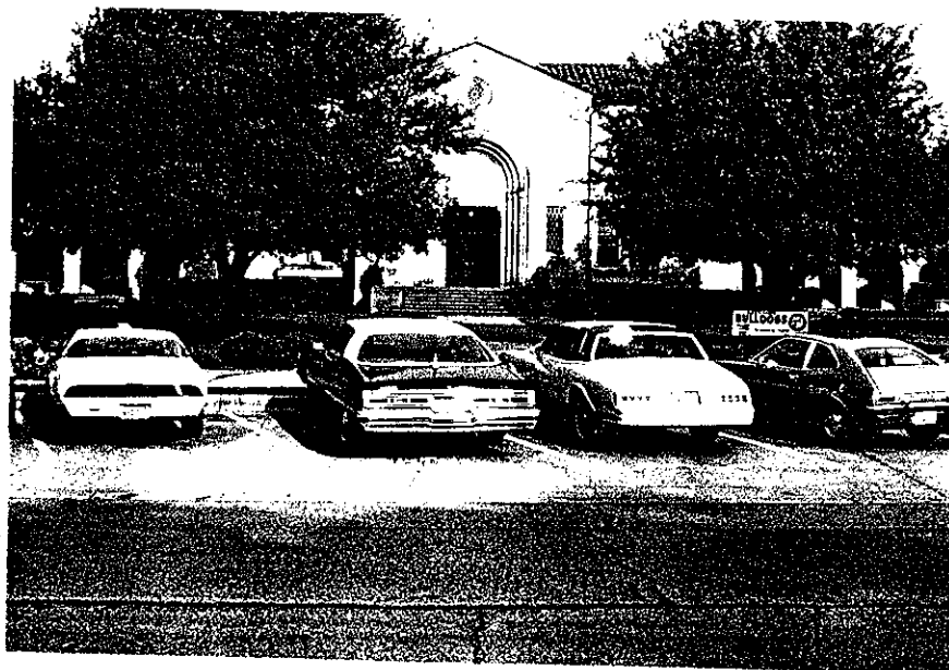
Kilgore High School 1986 Auditorium entrance
