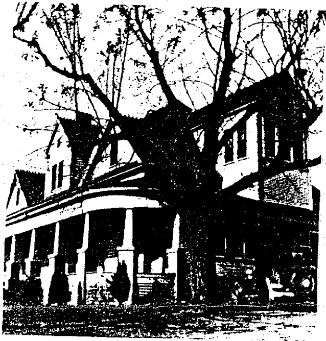
The Bumpus Home — For 50 years members of the Bumpus family have lived in this house which stands high on the hill at the corner of East Upshur and Center Streets. The family does not know when the house was built, but it has had several additions made to it through the years. The late Ray Bumpus bought the house from his mother, Mrs. W. E. Bumpus several years after his father's death.
