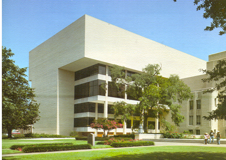
Gregg County Courthouse – West Wing – 1982
