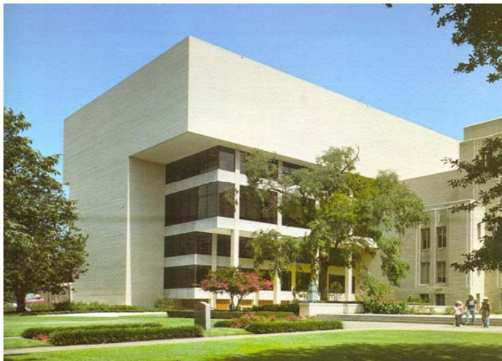
Gregg County Courthouse – West Wing – 1982
