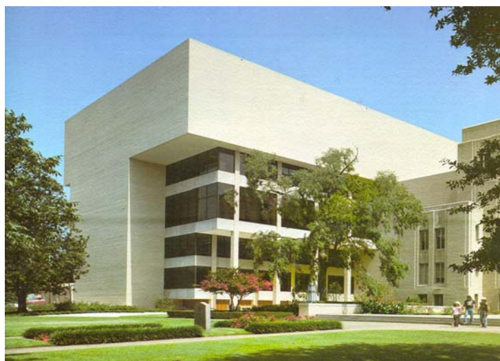
Gregg County Courthouse – West Wing - 1982
