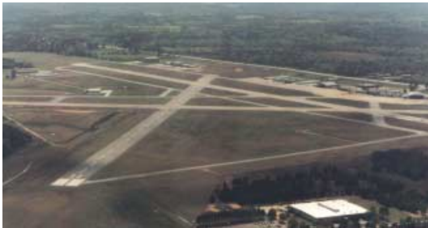
Aerial View of the Gregg County Airport
