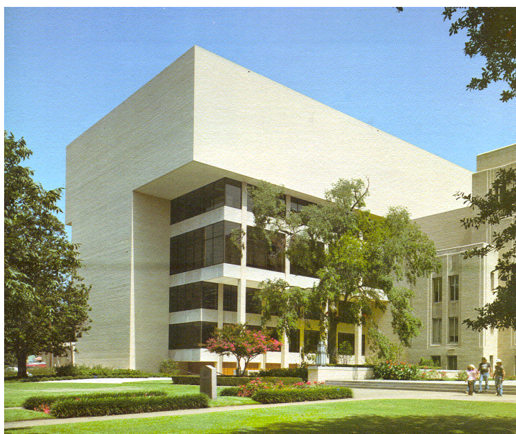
Gregg County Courthouse - West Wing - 1982
