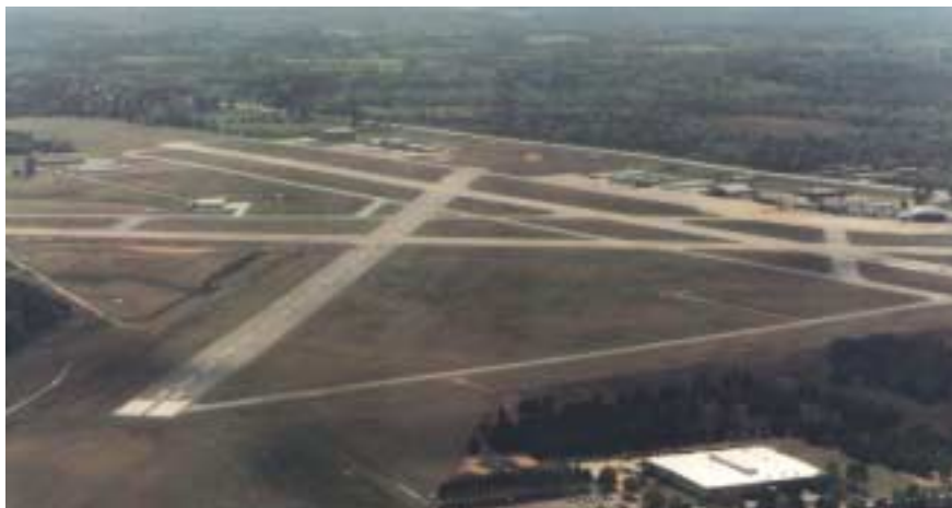
Aerial View of the Gregg County Airport
