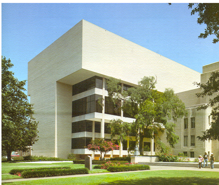
Gregg County Courthouse - West Wing - 1982
